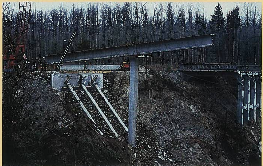
Fig. 8. A sloping-strut logging bridge, circa 1963.
