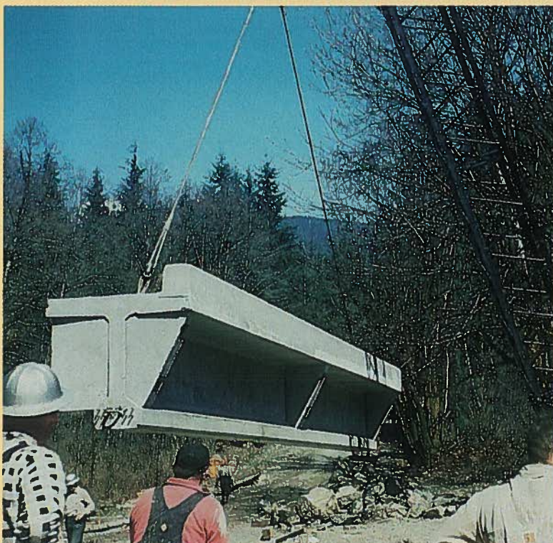
Fig. 4. A bulb-tee bridge for a logging road, circa 1955.
