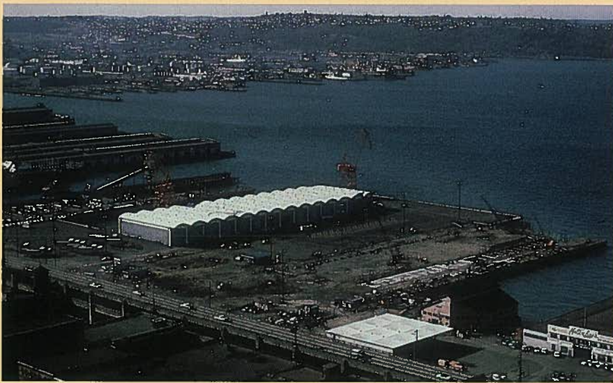
Fig. 14. Barrel-shell transit shed, Port of Seattle, circa 1963.
