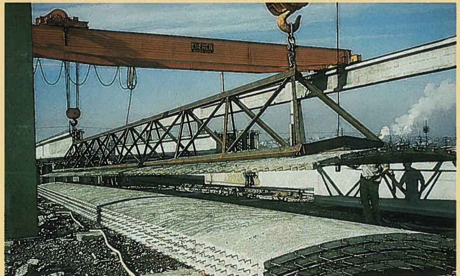
Fig. 13. A shell roof element handled by a steel truss strongback.
