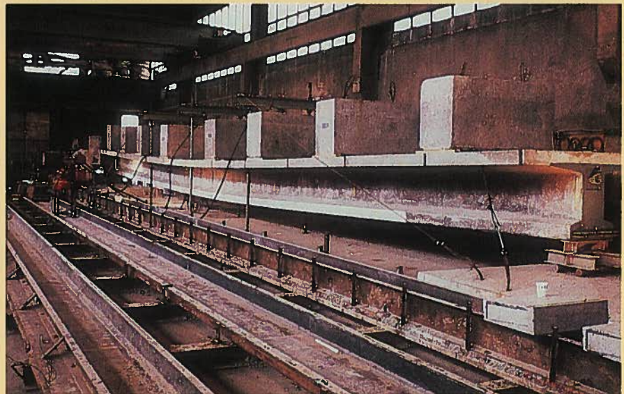
Fig. 7. A thin-flange prestressed concrete girder, circa 1959.
