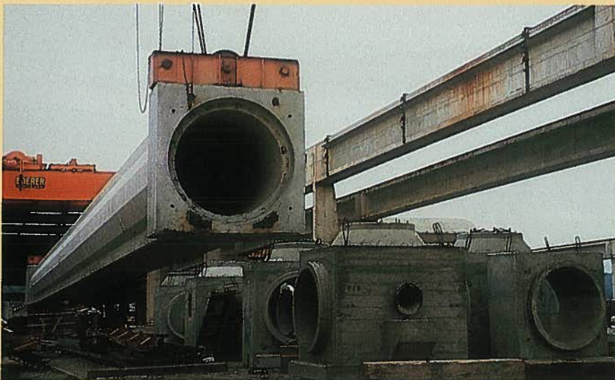
Fig. 16. An underwater sewer interceptor, Lake Washington, circa 1963.
