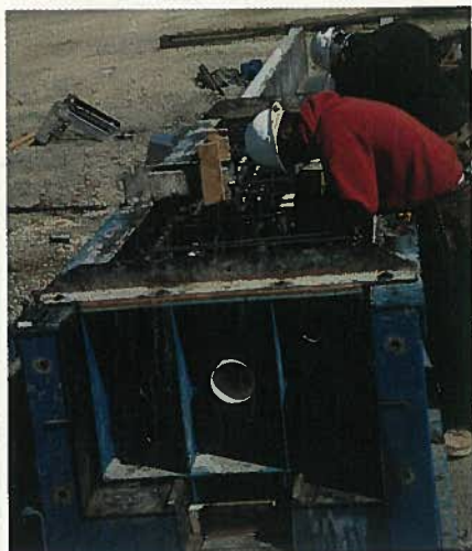
Setting up forms for beams.
