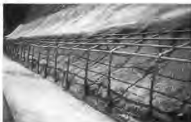
Installation of the C-BAR reinforcing bars in the Kennedy Mansion seawall.
