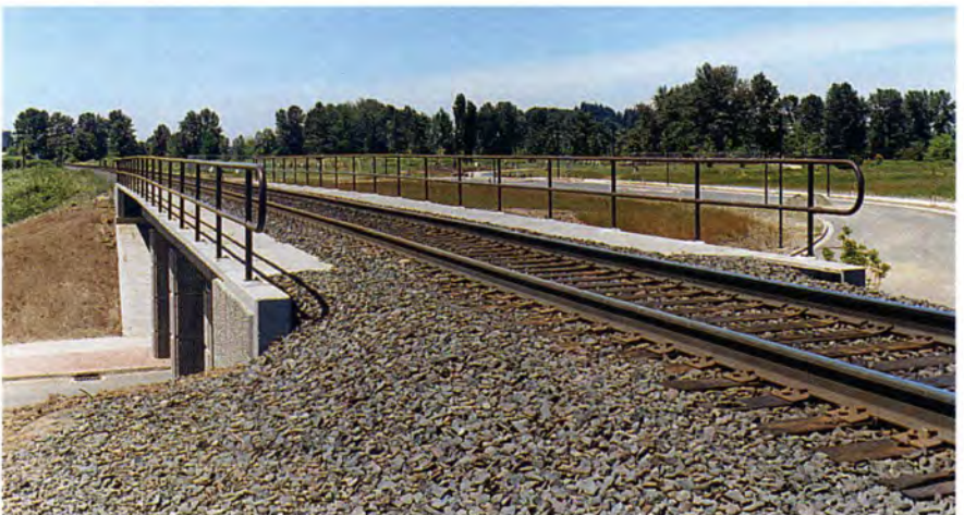
The 3 ft 10 in. (1.2 m) wide walkways were cast onto the box girders at the precasting plant after release of the prestressing.
