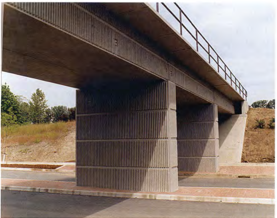
A "fractured fin" architectural finish was cast directly onto the precast box girders to match the finish on the cast-in-place coverings of the pile substructure.
