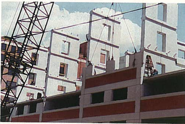
Installation of simulated brick faced precast concrete spandrel panels.
