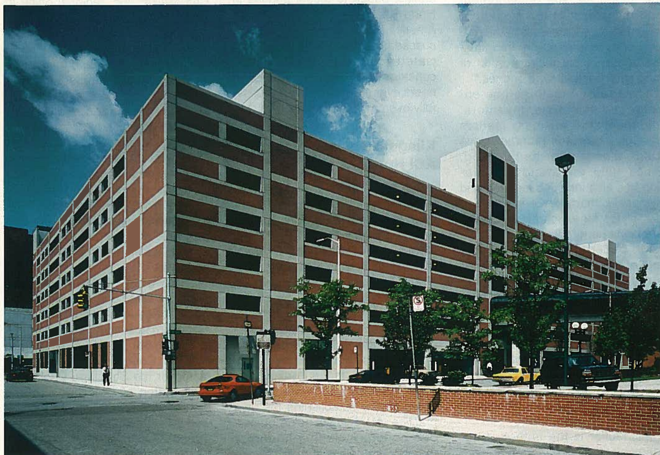
The Monroe Avenue Garage in downtown Detroit, Michigan, has a capacity of 1016 cars.
