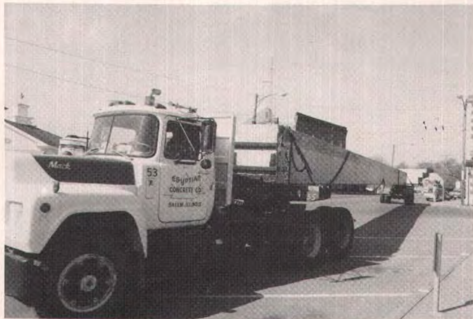
The logistics of transporting the precast prestressed concrete units presented very few problems.
