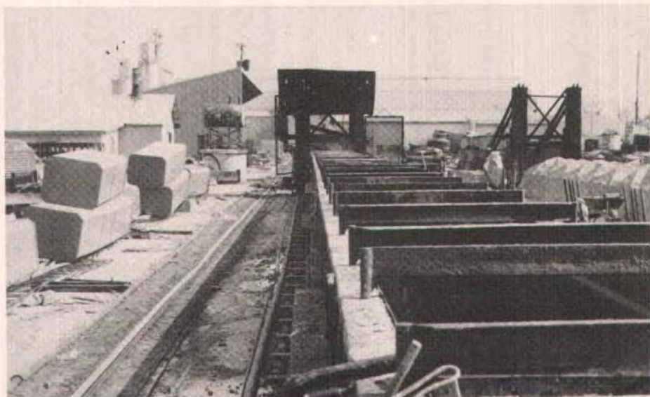
Form for deck beam with cardboard voids stacked at left.
