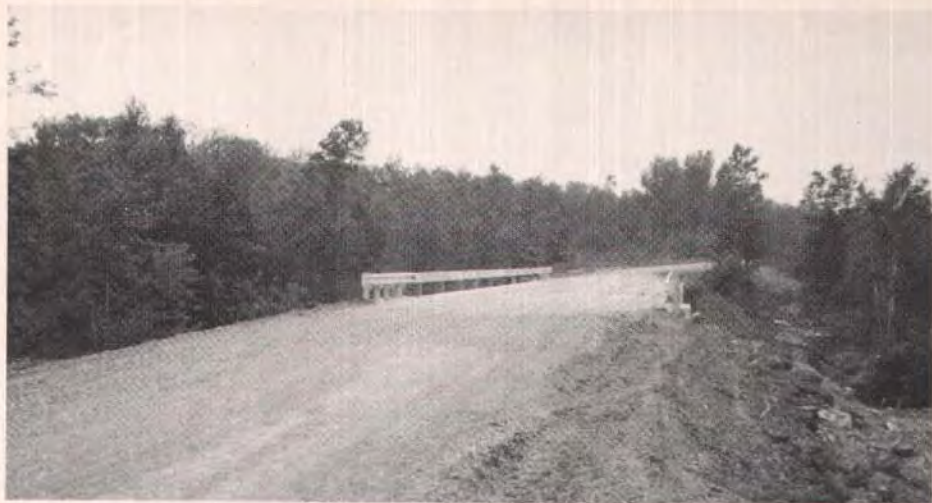
Structure with approach completed and open to traffic.
