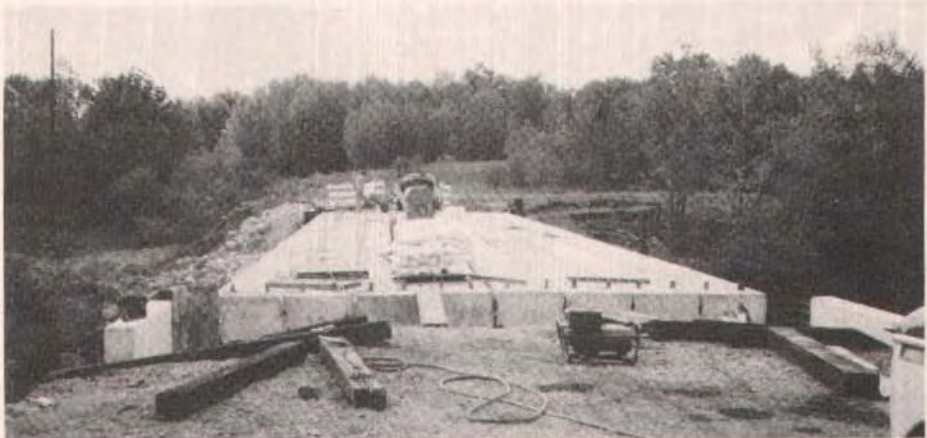
Deck beams in place, ready for grout.
