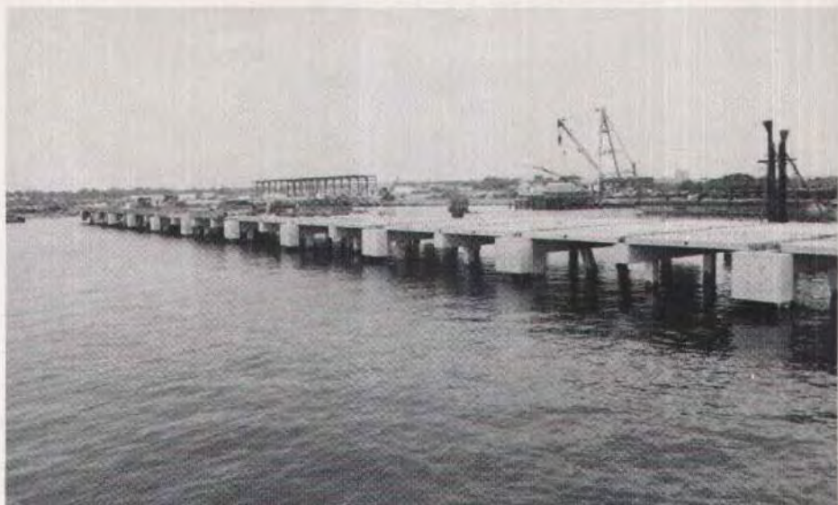
Fig. 2. Sea level view of pier.
