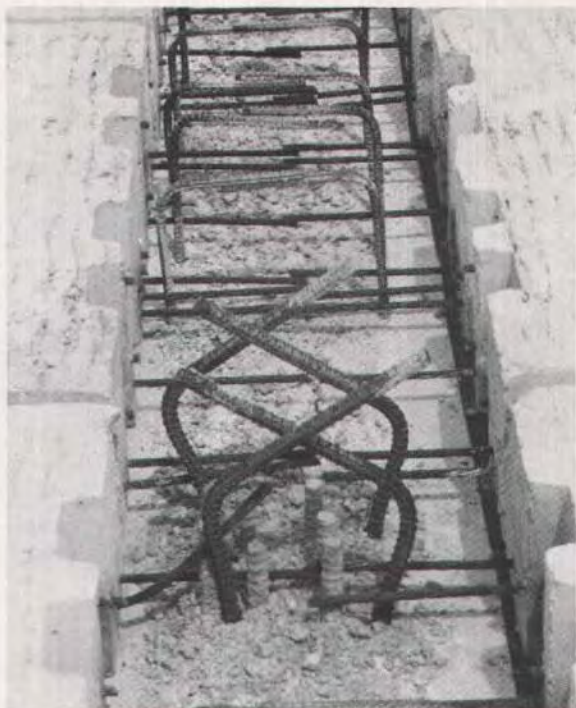
Fig. 4. Joint between precast planks over precast piers prior to placing of cast-in-place concrete.
