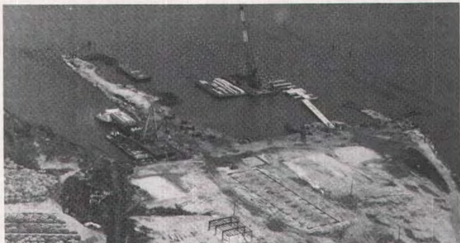
Fig. 8. Stage One: Construction after 40 days.
