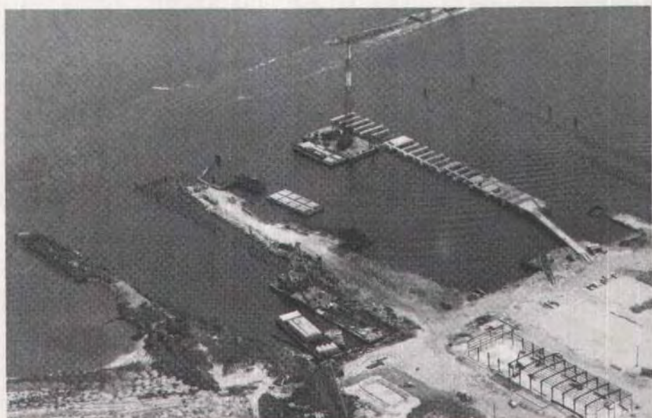
Fig. 9. Stage Two: Construction after 80 days.
