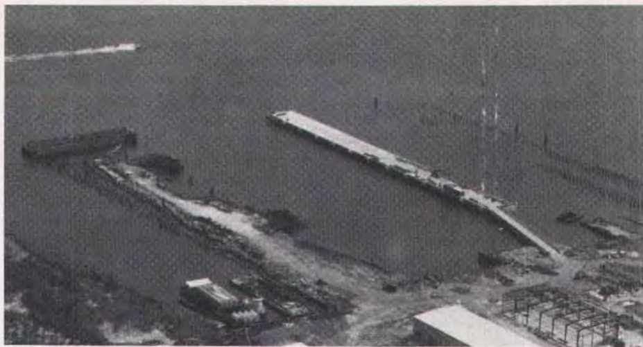
Fig. 10. Stage Three: Construction after 126 days.
