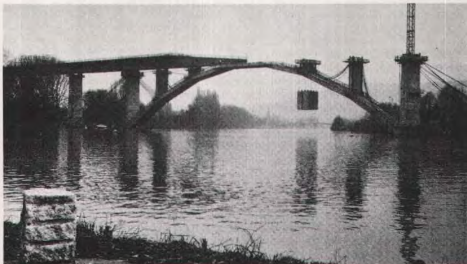
This prestressed concrete bridge being built over the Main River as part of a West German high speed rail network is reportedly setting a world record for the longest superstructure launched incrementally from one side. The Veitshöchheim Bridge cuts diagonally across the valley between two tunnels on the northern outskirts of Würzburg. By the time the last of 48 segments is cast, engineers will be pushing an unprecedented 4,143 ft (1268.8 m) of deck girder, weighing 40,000 tons (36,288 t) over teflon bearings atop 28 piers. Above: Long girder launch passes over arch as cables restrain river piers against jacking forces.
