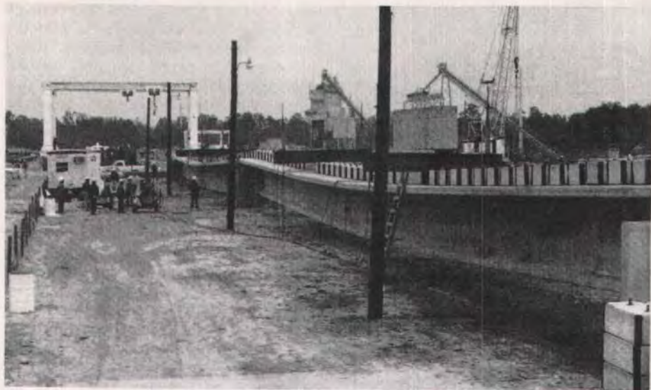
Prestressed bulb tee is loaded to failure in what is believed to be a test of the largest such girder ever.
