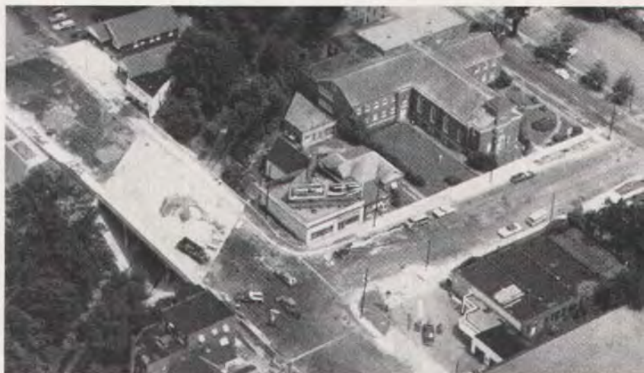
Fig. 8. Aerial view of the new bridge and roadway (during construction).
