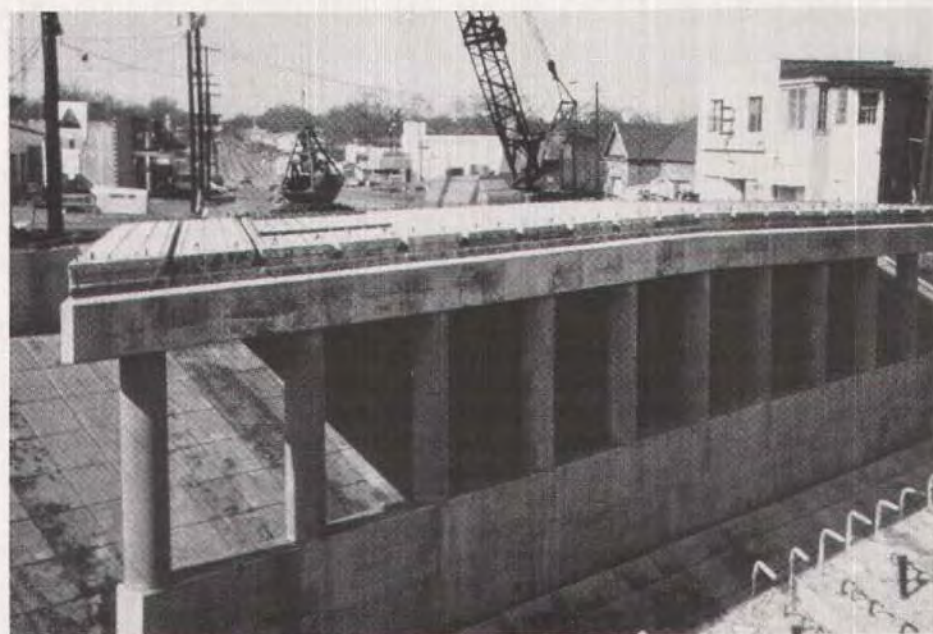
Fig. 3. 35 ft (10.7 m) span on the west side of new bridge.
