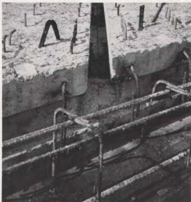
Fig. 4. Adjoining slabs prior to placement of reinforced concrete overlay.
