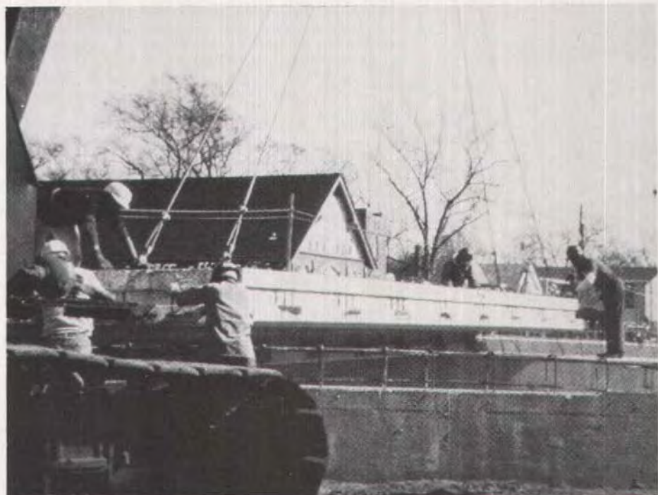
Fig. 2. Placement of voided slabs.
