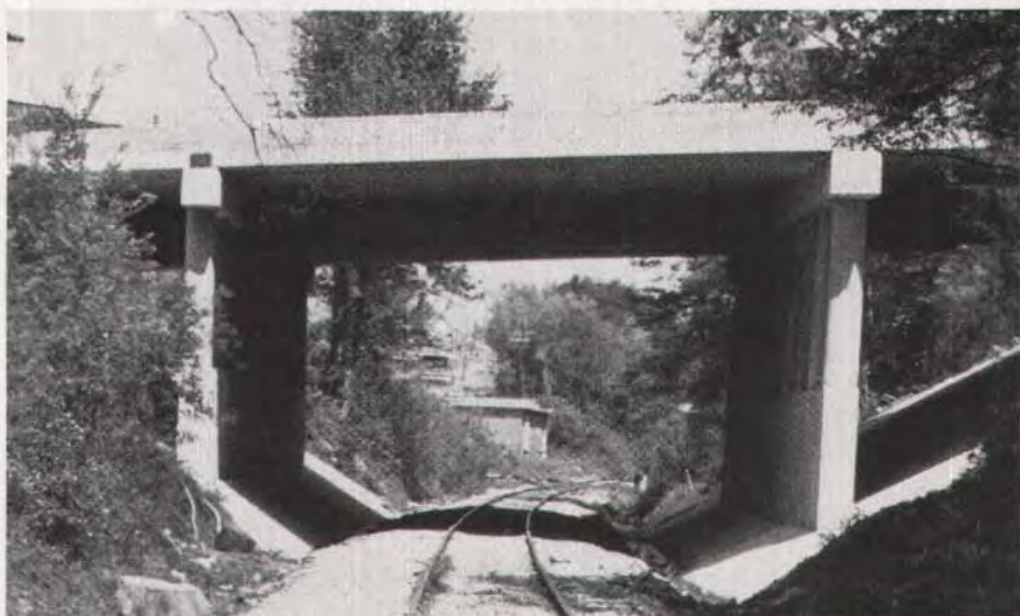
Fig. 6. Improved clearances with new precast prestressed bridge.
