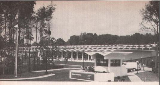
The building system also provides two other advantages: the shape of the Y beams helps diffuse noise in the plant, and the extensive use of precast concrete provides a fire-resistant plant structure.
