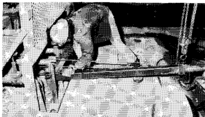
Fig. 12. Here chalk marks are made on the ram to check elongation. When initially tensioning the strand, "release slippage" must be accounted for at the live end. This is the distance the strand slips back into the chuck until the inserts fully hold the strand in position. During final tensioning, chuck slippage at both the dead and live ends must be considered when cross-checking strand tension with elongation.
