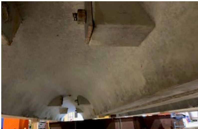
Figure 2 – Bolt Connections between Arch Beams
