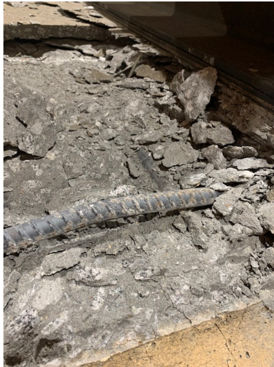
Figure 17 – Buckled Compression Steel
