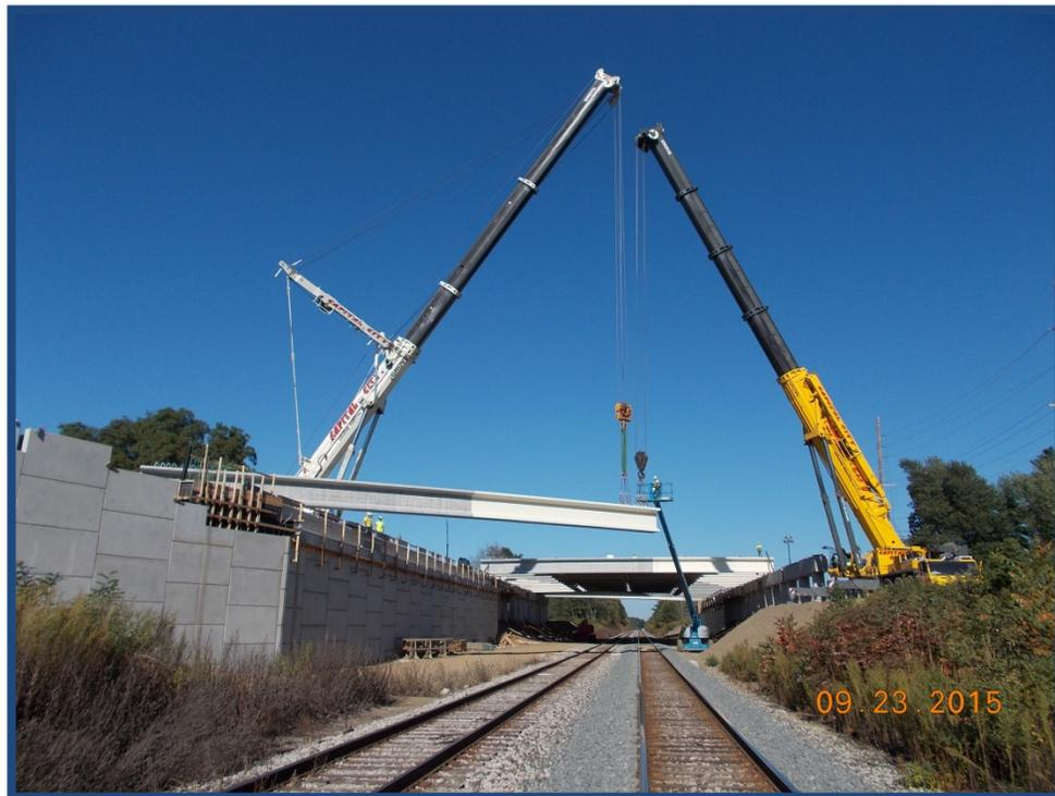
*Figure 6: Beam Erection*
