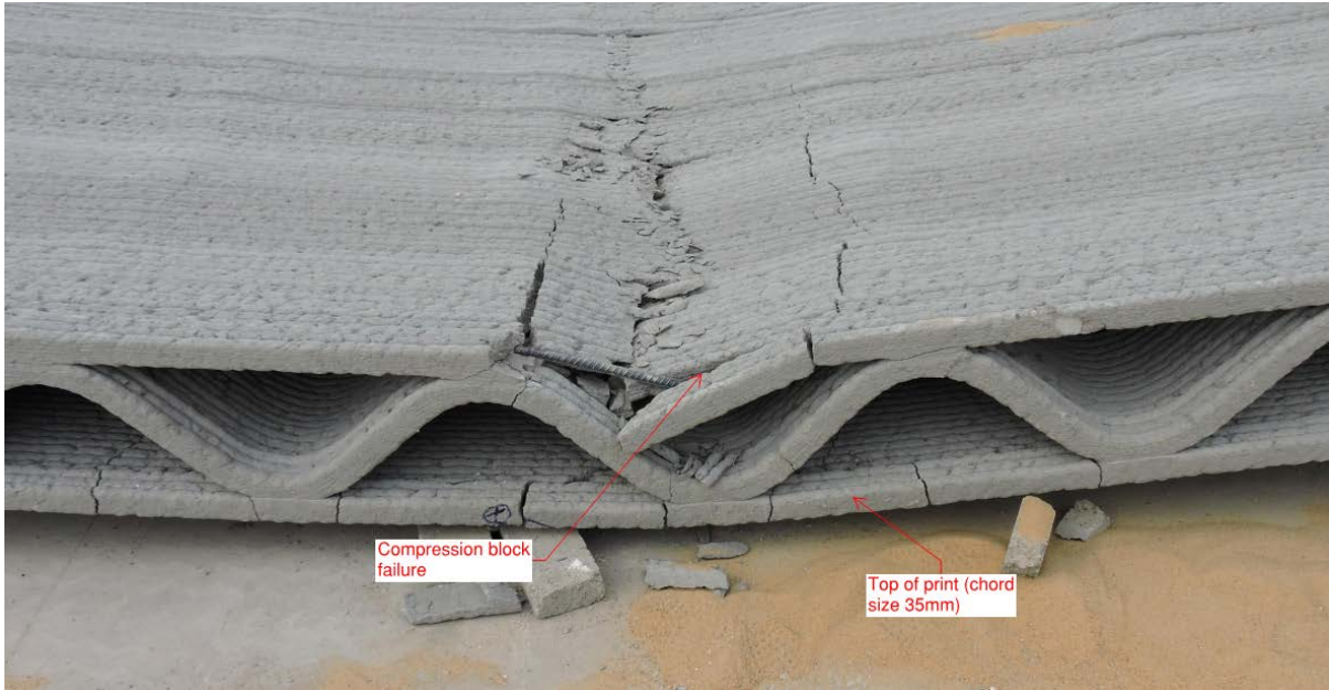
Fig. 11: Failure mechanism at top of the print.
