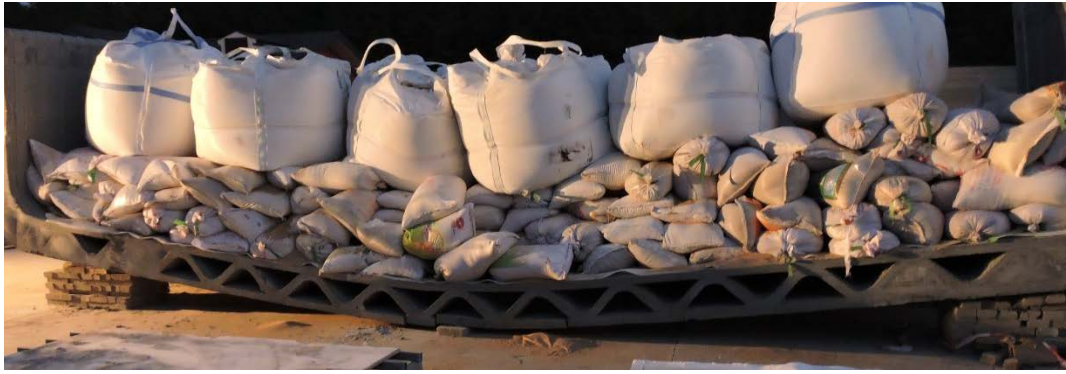
Fig. 9: 3D printed bottom cassette at the failure testing load
