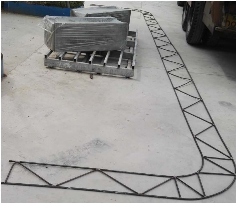
Fig. 6: Prefabricated rebar steel truss
