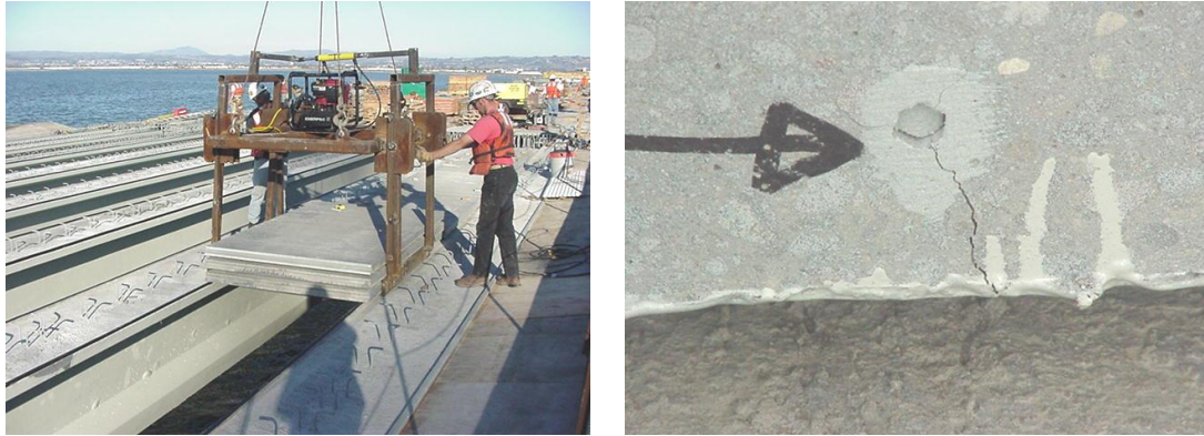
a) Placement of Deck Panel
