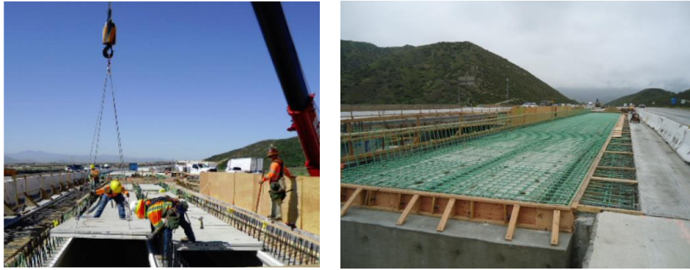
a) Placement of Deck Panel
