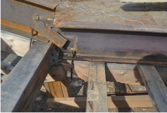
Fig. 11 Damaged joists and welds
