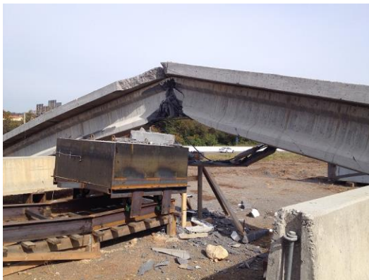
Fig. 10 Beam after impact
