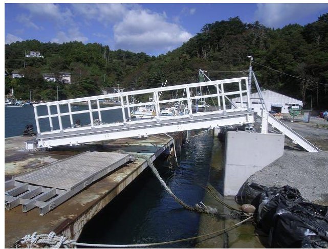
(b) Completion of GFRP-UHPFRC pedestrian bridge connecting a pontoon and a concrete pier
