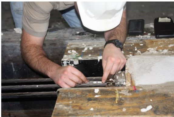
Figure 3. Measurement of strand end slip using steel block clamped to strand and depth micrometer
