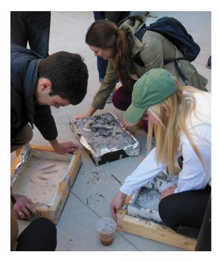
Fig. 1 Architecture students at Miami University working to release precast concrete panels from their formwork.
