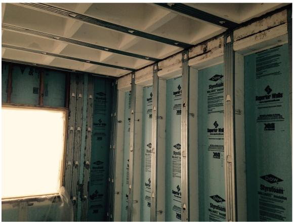
Figure 16: After the decision was made to investigate a precast concrete system, the precast company suggested a system to the design team that would include insulated and studded panels for both floor and walls.
