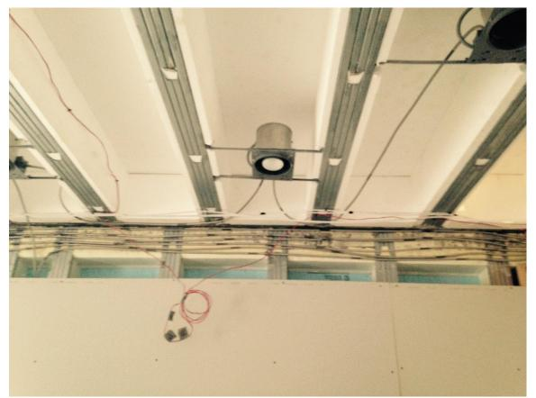
Figure 17: The wall and floor panels permit the running of plumbing and electrical systems within their assembly dimension. The piping and wiring were coordinated between the architect and precast company.
