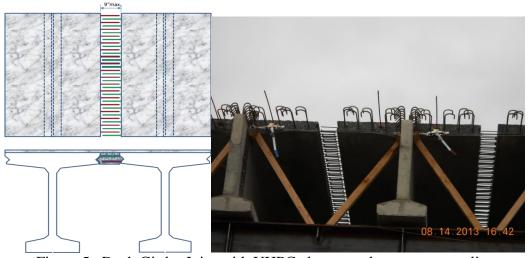
Figure 5. Deck Girder Joint with UHPC closure and non-contact splice
