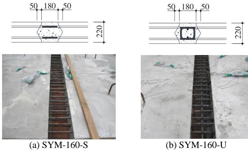
Fig. 8 Geometry of the precast deck joint and bar details (Note: 1 in. = 25.4 mm)
