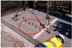
Fig. 2 Predesigned shear pockets in the base slab for anchor embedment
