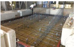
Fig. 10 Fabrication process of wall face and counterforts showing extended L-bars
