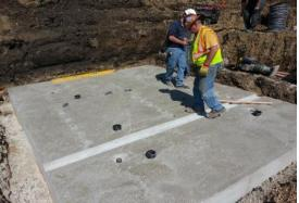
Fig. 12 Finishing the erection of the base slab
