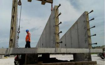
Fig. 1 Anchors extended from the counterfort
