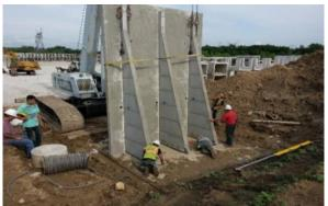
Fig. 13 Final assembly of TPCCRW
