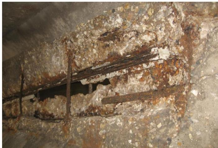
Figure 1. Strand and rebar deterioration in US 45 bridge in Milwaukee.
