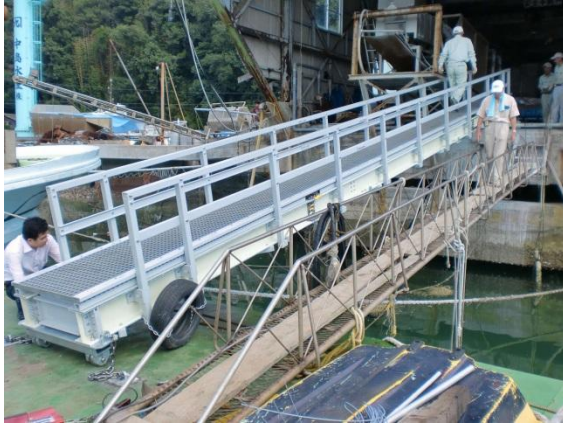
(a) Newly constructed FRP bridge using HFRP I-girders
