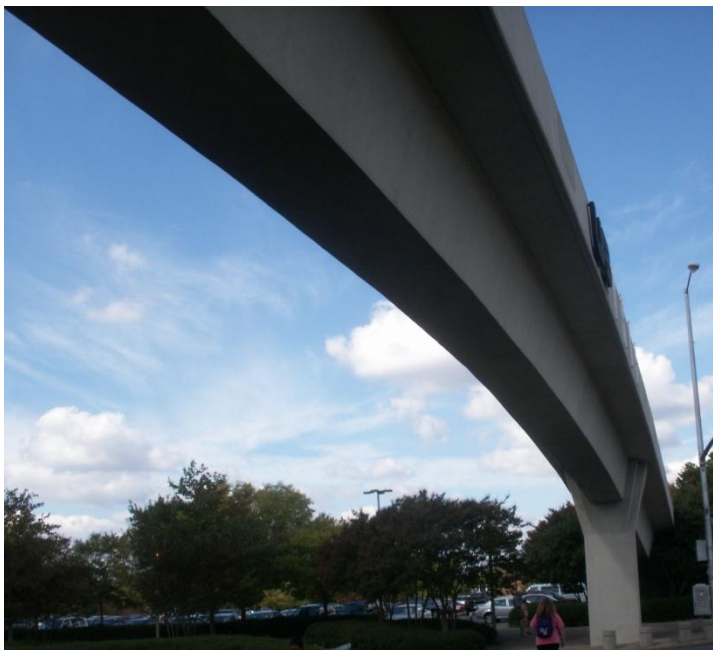
Fig 8 Pedestrian bridge over University Blvd. at UAB
