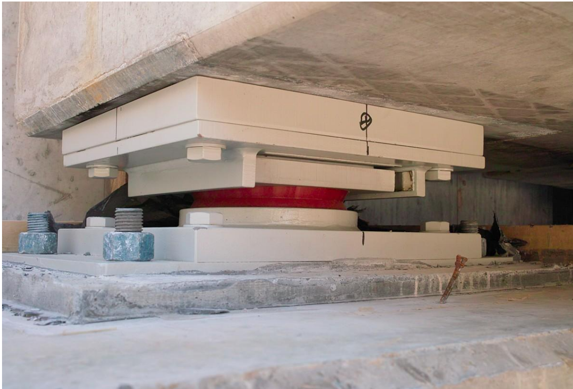
Fig. 10 Disk bearing with replaceability detail
