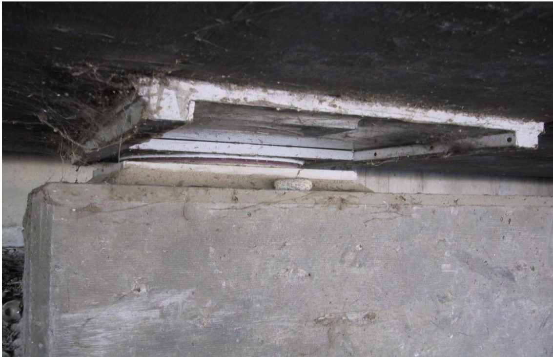
Fig. 4 Thirty-five year old disk bearing on the Pasco Kennewick Bridge
