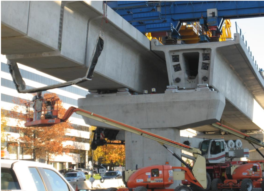
Fig. 12 Disk Bearings supporting the concrete segments on the Dulles Project
