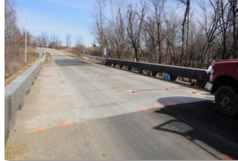
**Figure 8:** Load Paths Marked on Bridge Deck
