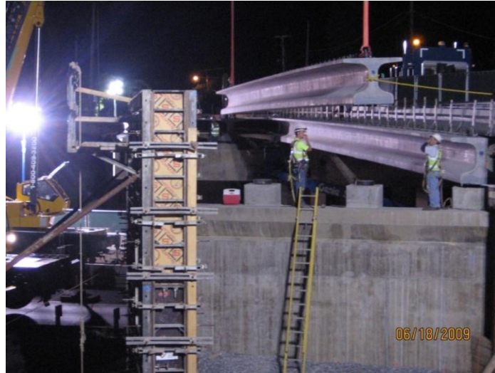
Erection of Northerly Span #1 Girders, Showing Back of Abutment #1
