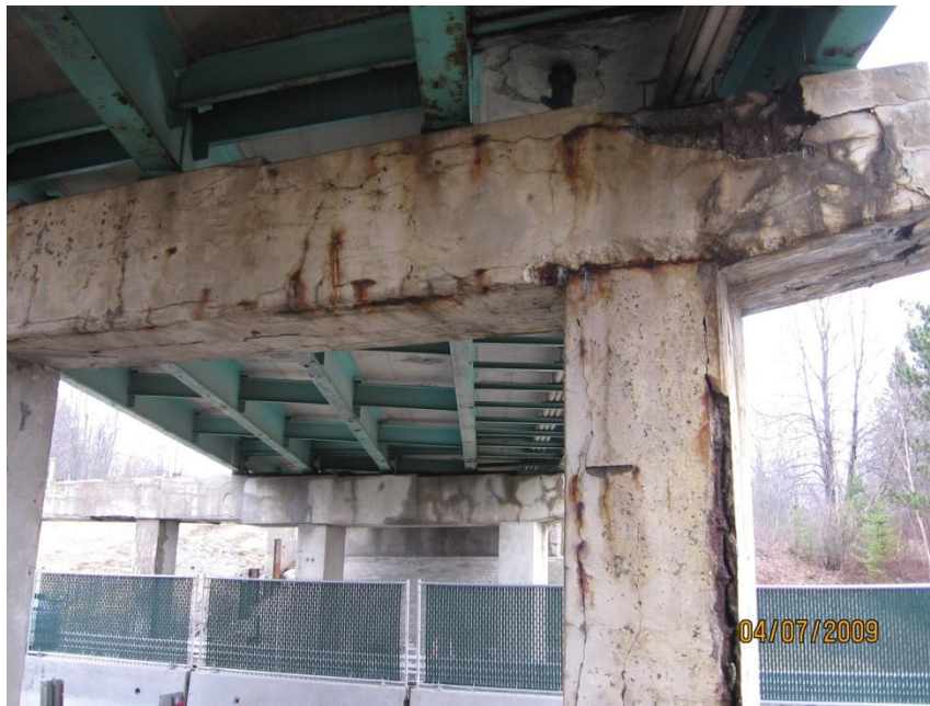
Underneath Previous Bridge w/ Central Pier in Foreground
