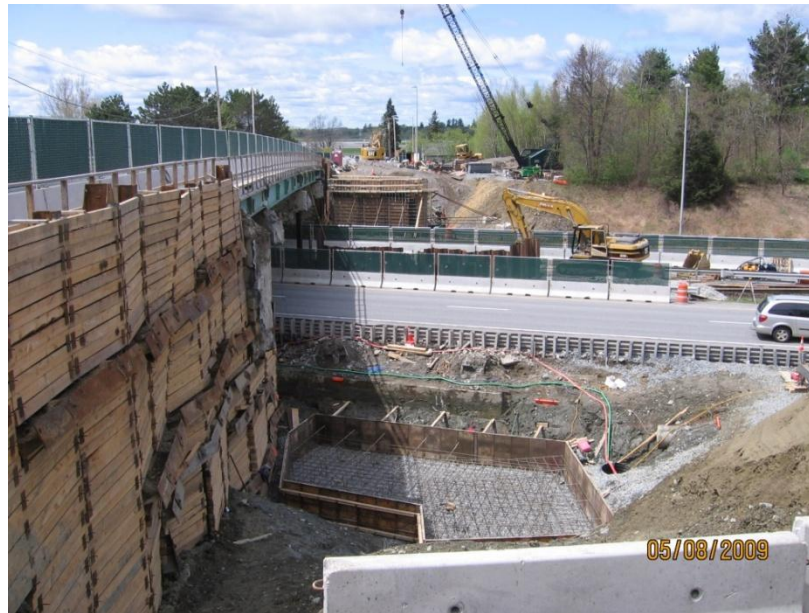
Looking Westerly with North Half of Previous Bridge Removed
