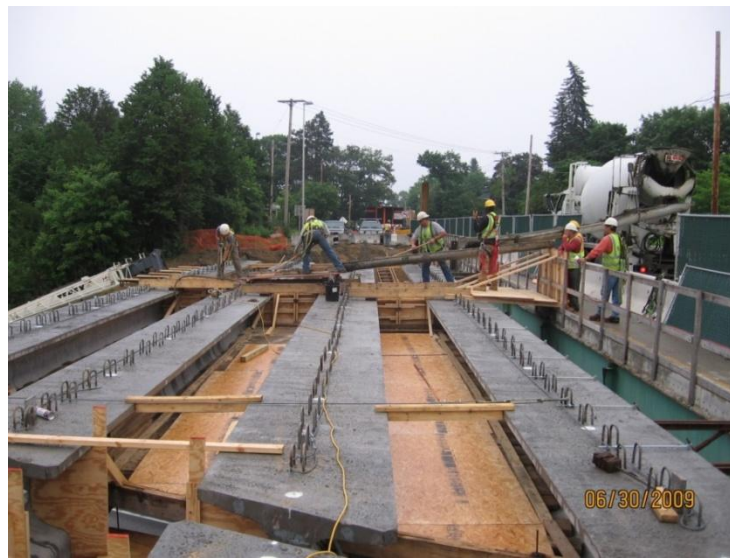
Intermediate Diaphragm Placement w/ Beams Awaiting Pier Splice
