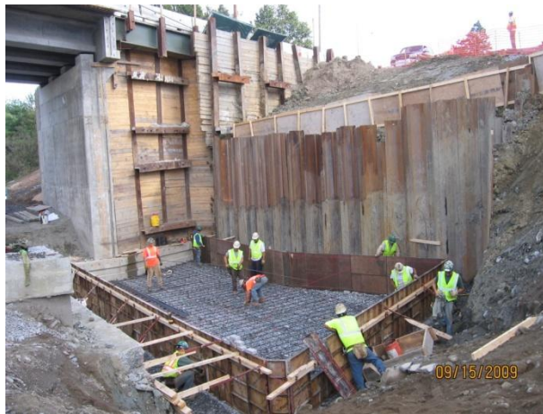
Stage Construction of 2 nd Half of Abutment #2 Footing – SE Corner
