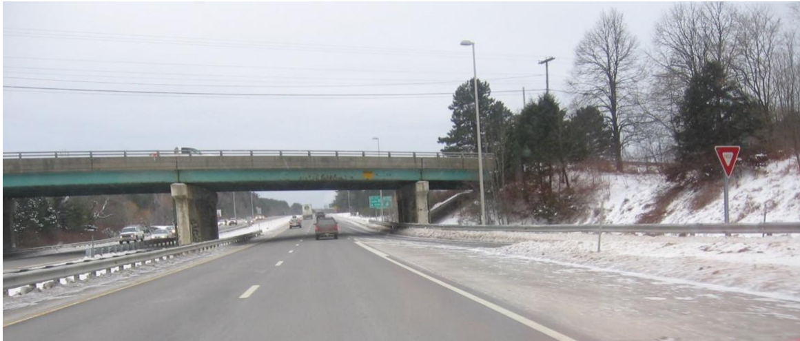
Looking Southerly at West Half of the Previously Existing Bridge
