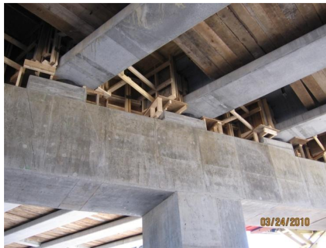
Framing for Formwork of the Pier Continuity Collars and Diaphragm
