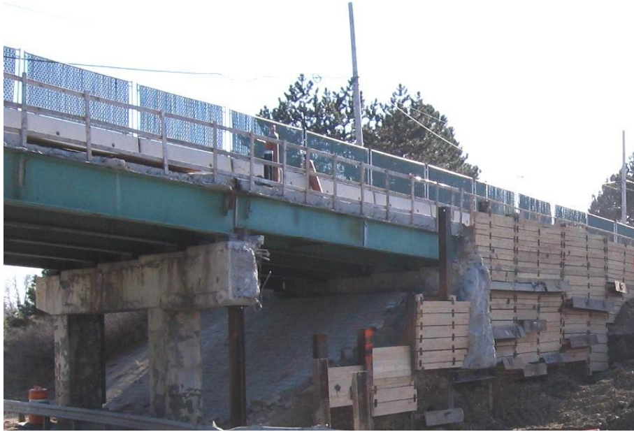
Half Existing Bridge Supported on Half of Westerly Pier
