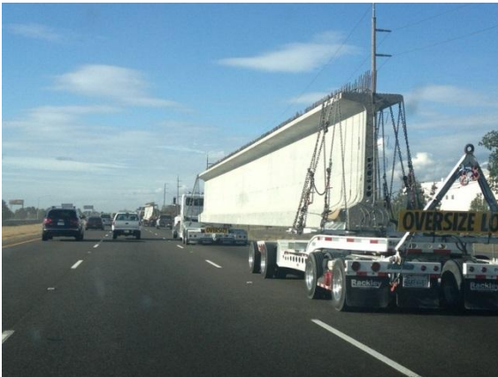
Fig. 18: Girder transportation
