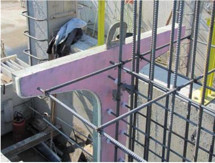
Fig. 9: Paste retarder applied to end forms
