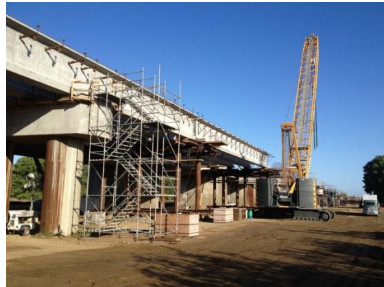
Fig. 21: Daytime view of erected girders
