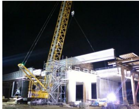
Fig. 19: Girder erection
