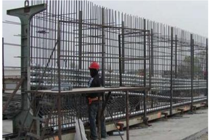
Fig. 8: Post-tensioning ducts positioning
