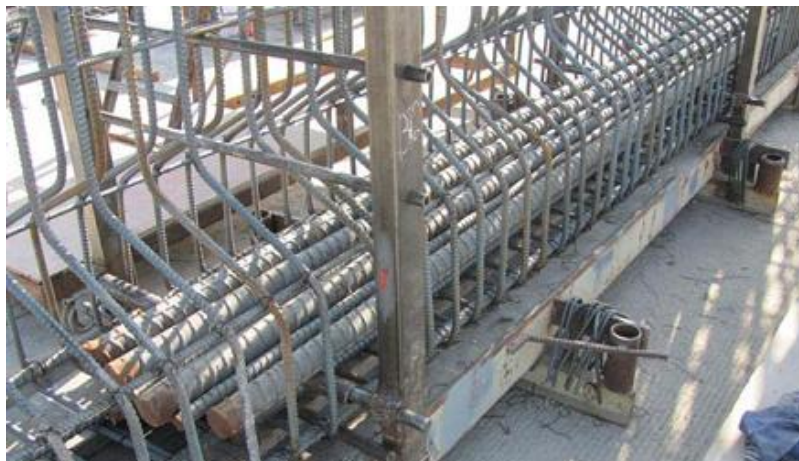
Fig. 15: Bottom flange additional reinforcement
