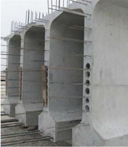
Fig. 7: Post-tensioning ducts
