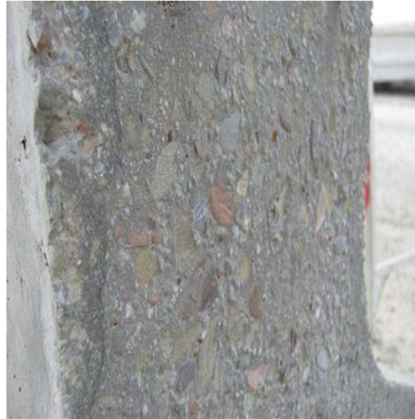
Fig. 17: Sandblasted surface profile
