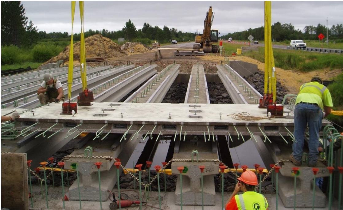
Figure 6 Deck Panel Installation
