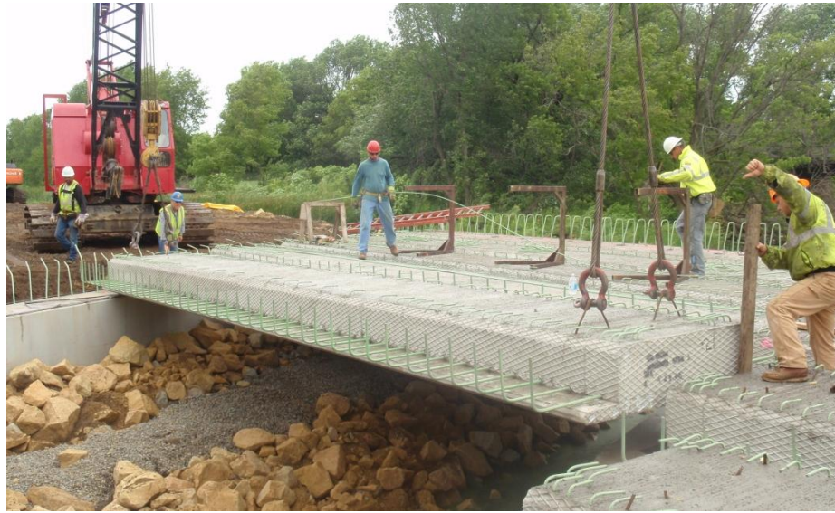
Figure 3 Erection of Inverted Tee Sections
