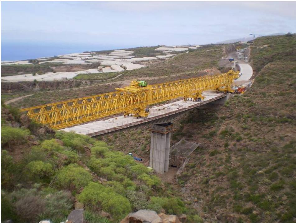
Figure 13: In Situ Casting.
