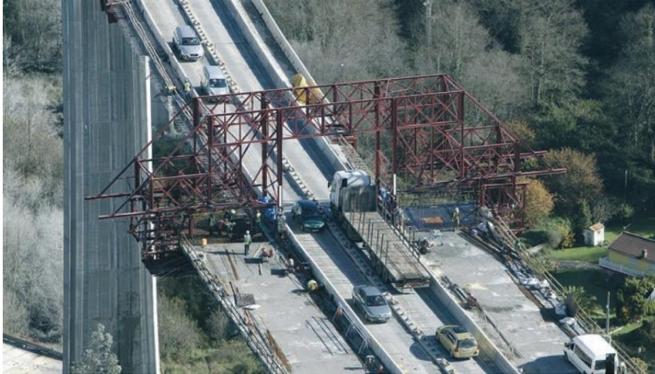
Figure 12: Alternative solution. Example of Secondary Gantries with Elaborate Falsework<sup>3</sup>
