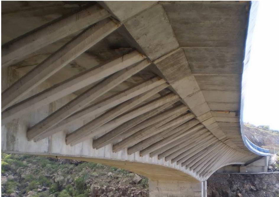
Figure 4: View of the Longitudinal Rib of the Overhang Support
