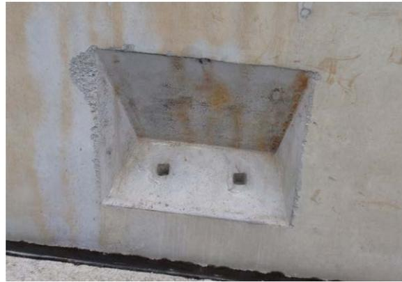
Figure 5: Strut Support Recess
