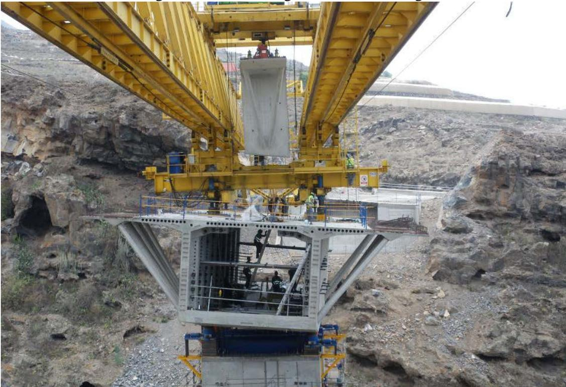
Figure 11: Placement of the Precast Segments
