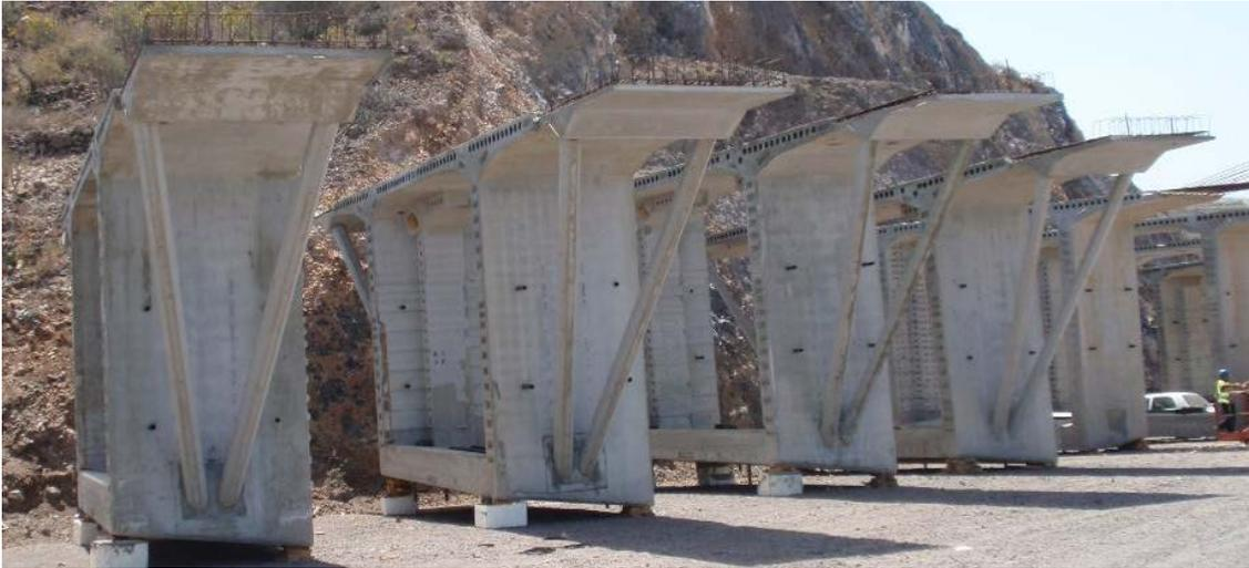
Figure 10: Stacked Segments in the Casting Yard
