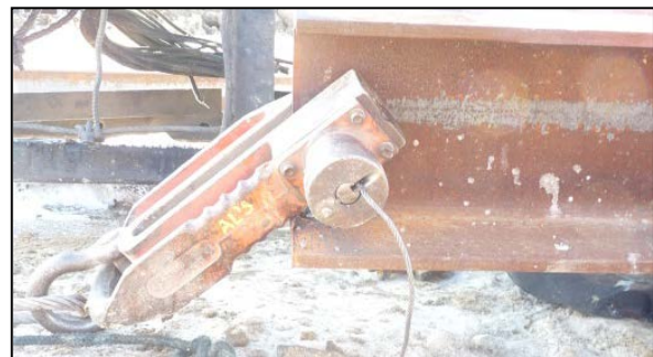
Fig. 15 Pickup Point for Steel Piles
