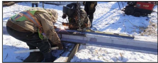
Fig. 5 Splicing UHPC Test Pile Horizontally on the Ground
