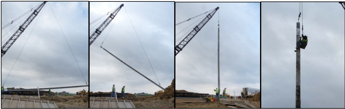
Fig. 17 Stages of the Pickup of UW1-2
