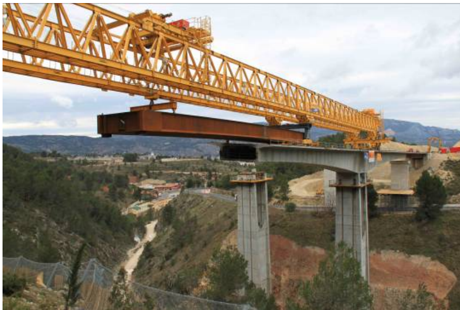
Fig. 11: Launching the south box beam to the abutment.
