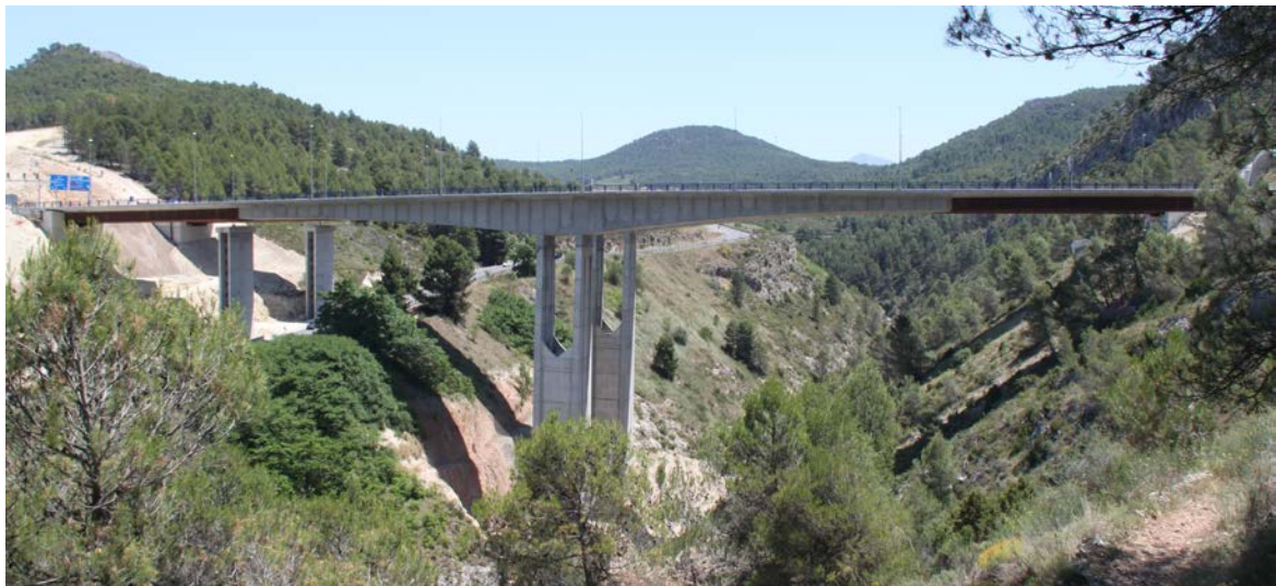
Fig. 16: Bridge finished (before demolishing the provisional piers).
