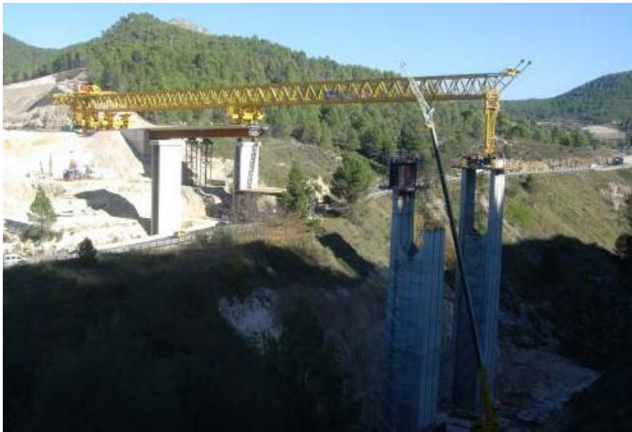
Fig. 7: Launching to the permanent pier.
