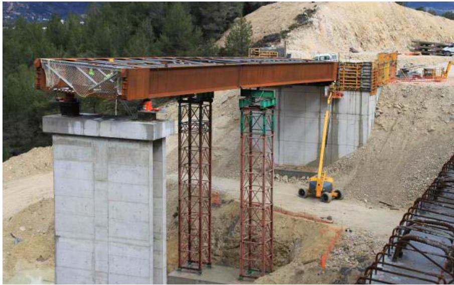
Fig. 6: Assembly of the north steel beam.
