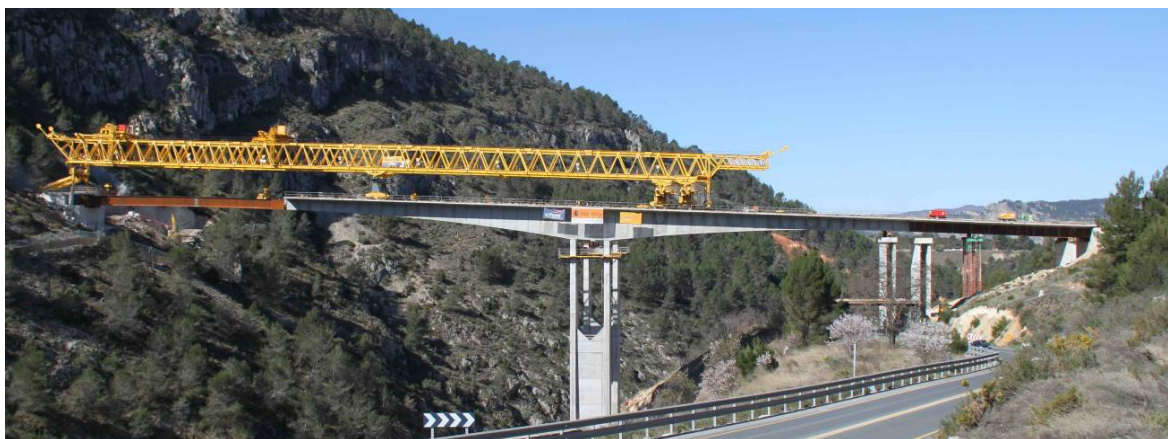
Fig. 3: View of the viaduct under construction (placing south steel beam).
