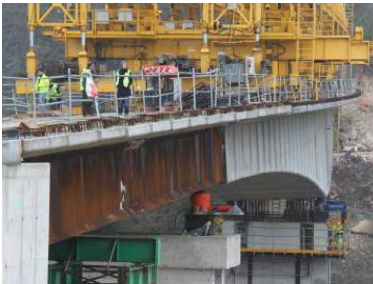
Fig. 9: Orientation of the T120 and the north composite beam.
