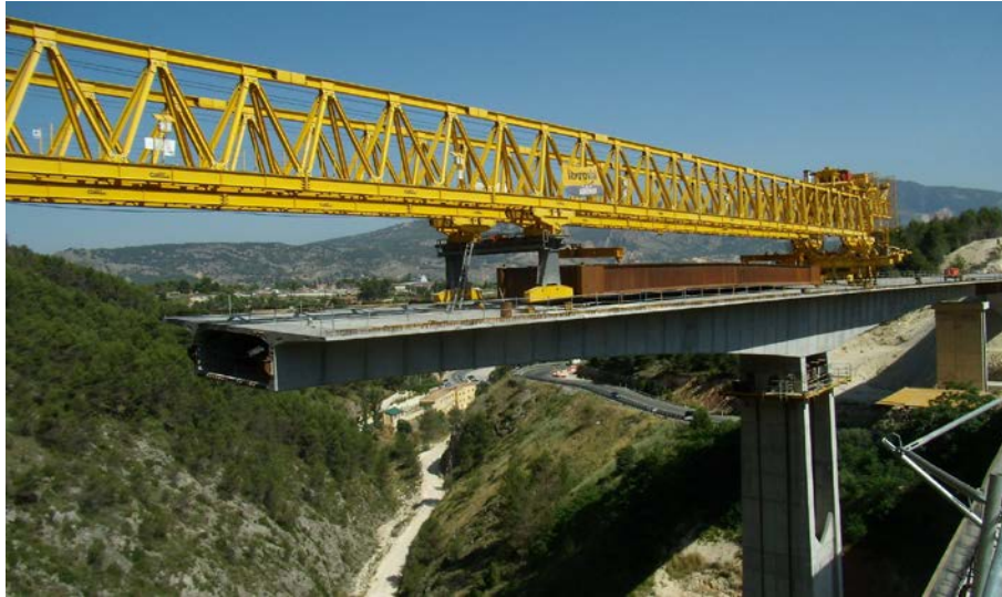
Fig. 10: Advance of south box beam over the deck.
