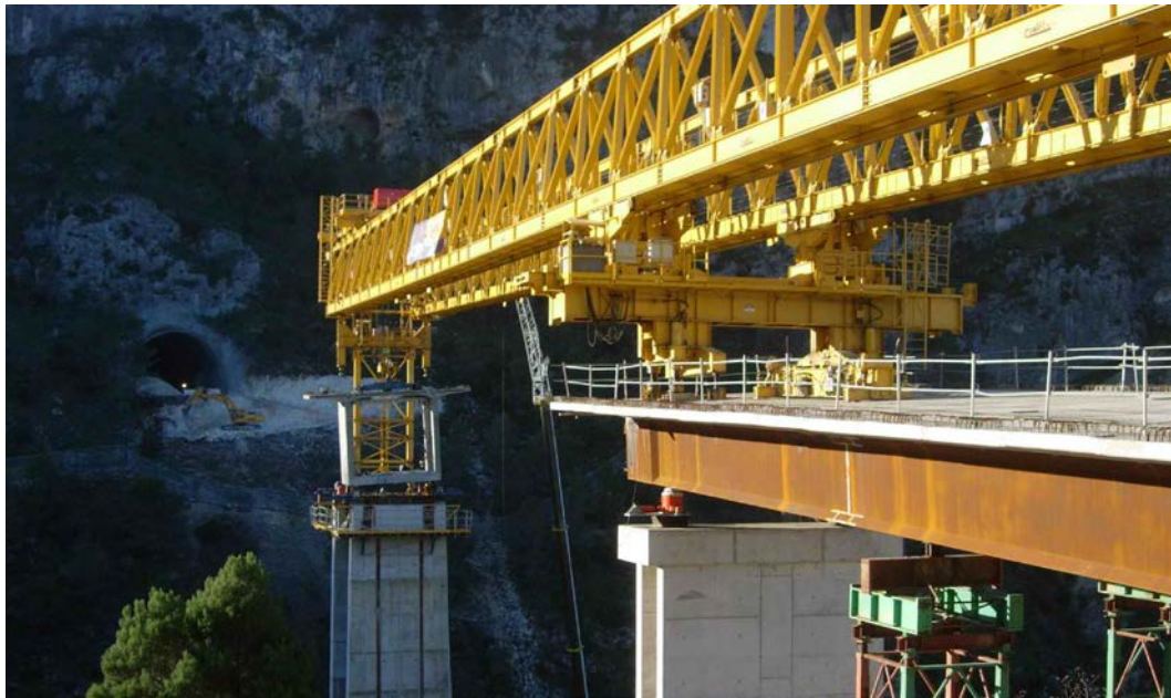
Fig. 8: Placing “cero” segment.
