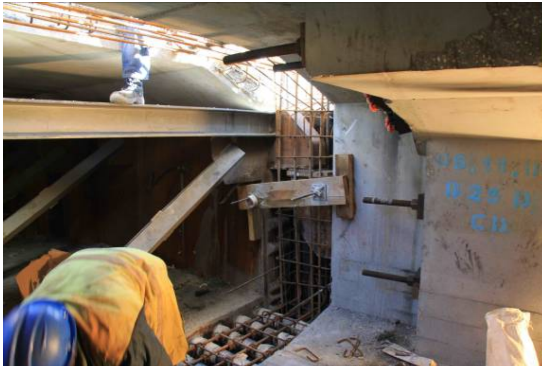
Fig. 15: Connecting the T120-section and north box beam.
