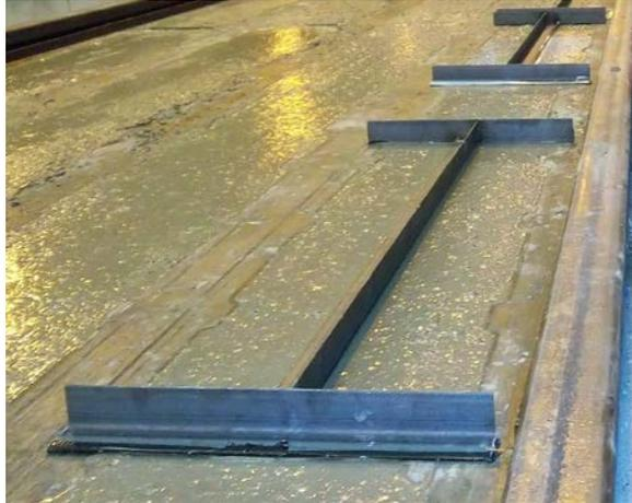
**Figure 17. Steel bars cast in fresh concrete**
