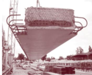
Fig. 2 Poutre-Dalle system observed in France during the 2004 Scanning Tour (Picture courtesy of Federal Highway Administration (FHWA)<sup>1</sup>)
