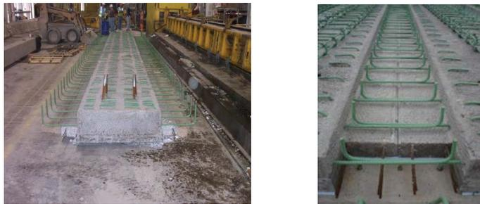
Fig. 3 Precast Inverted T-beam used by the Minnesota Department of Transportation (MnDOT) (Picture courtesy of MnDOT<sup>5</sup>). Picture on the left shows as a typical precast inverted T-beam while picture on the right shows the field installation of the precast inverted T-beams side by side.
