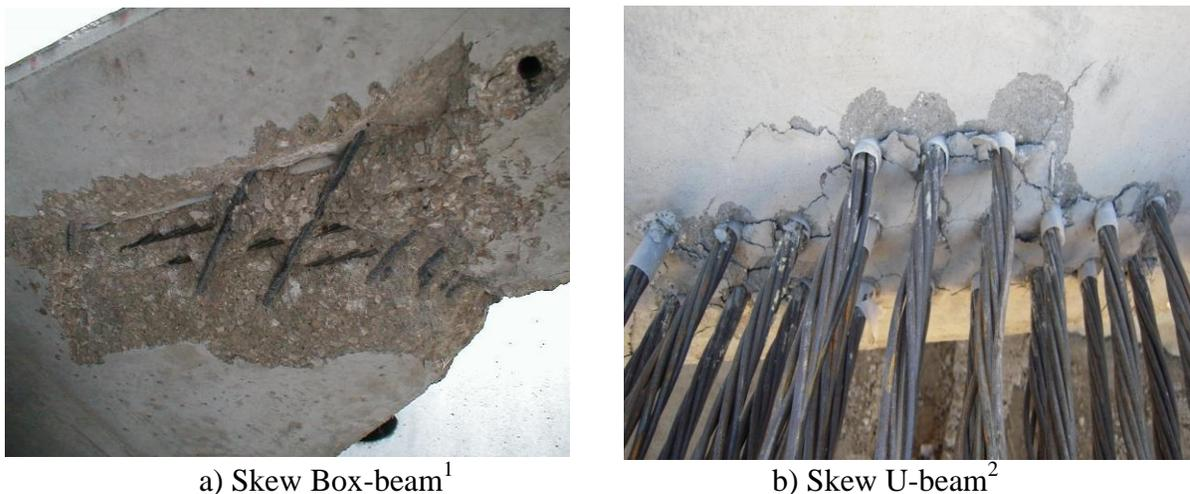
Fig. 1 Damage at beam ends of prestressed bridge girders during production
