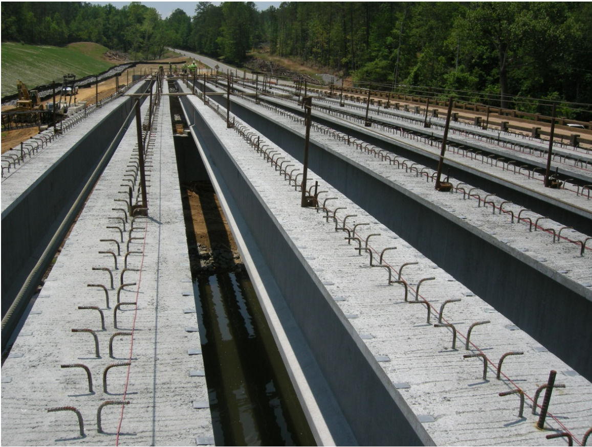
Fig. 1 Construction of precast, prestressed bridge over Hillabee Creek in Alexander City, AL
