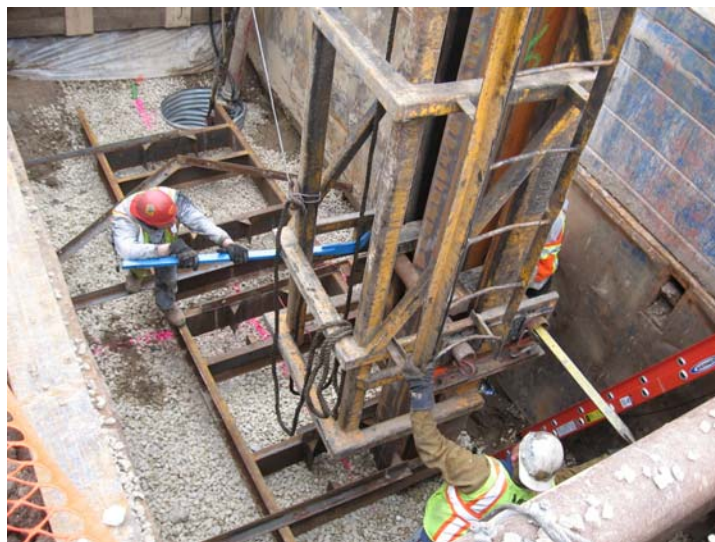
Fig. 5 Driving Pile at Pier
