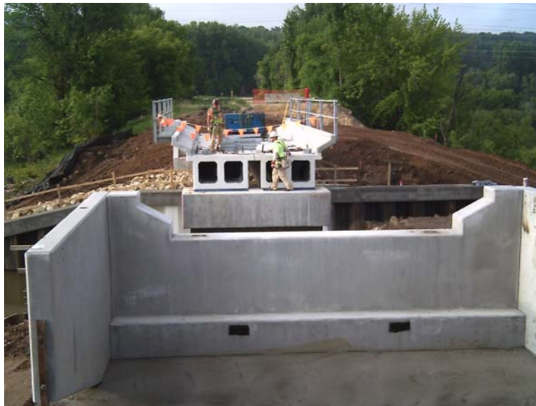
Fig. 6 Railroad Bridge Precast/Prestress Box Beam Installation
