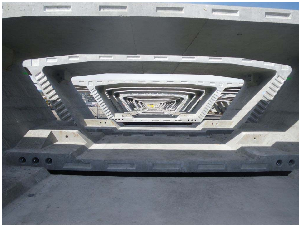
Fig. 10 Casting Yard, Typical Segment Storage
