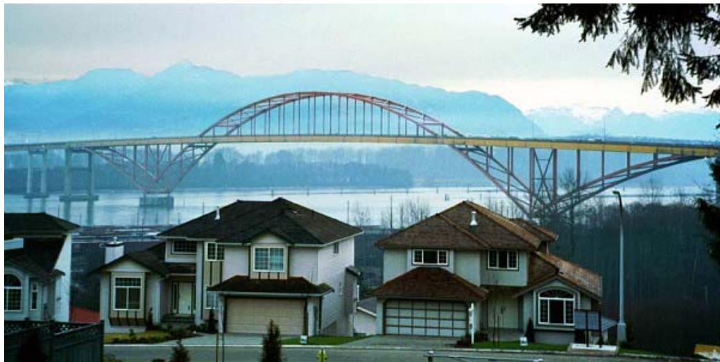
Fig. 2 Existing Port Mann Bridge
