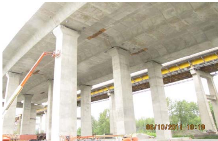
Fig. 23 Typical Pier Segment being transported
