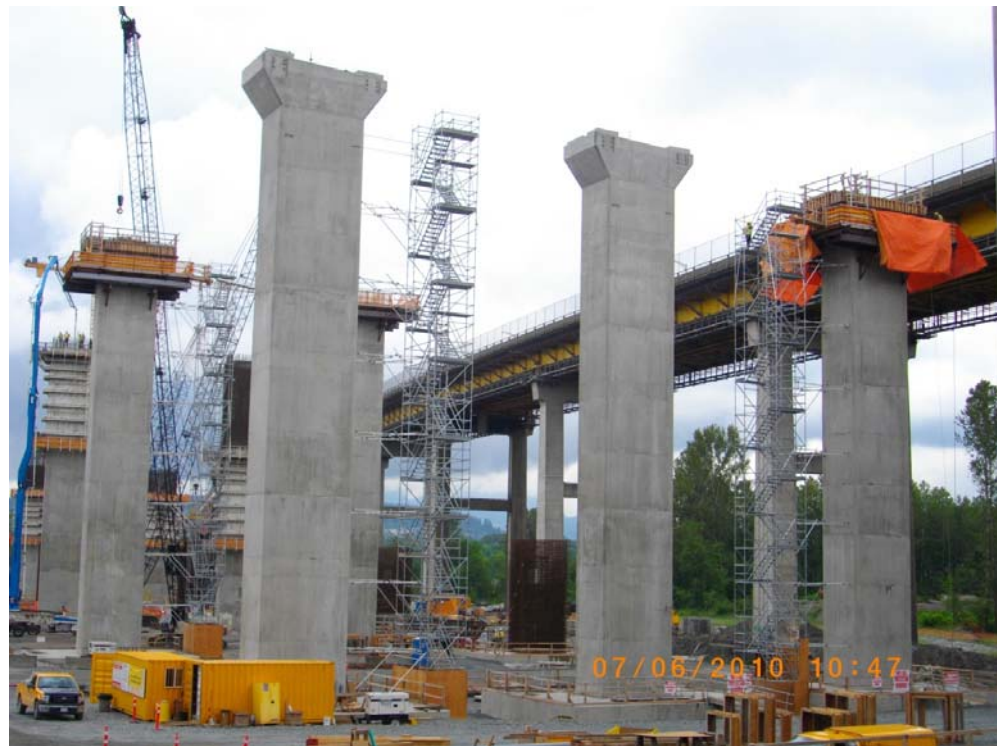
Fig. 21 Site Photo of Column Construction
