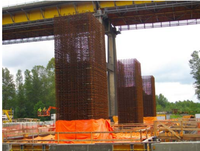
Fig. 22 Pier Reinforcement
