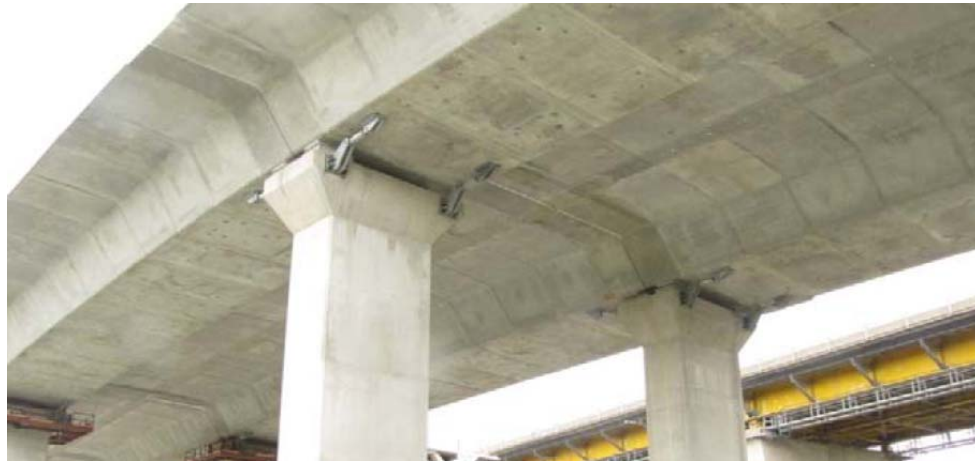
Fig. 15 Start of Cantilever Construction
