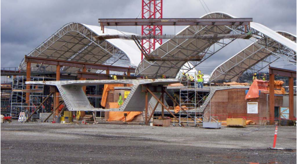
Fig. 9 Casting Yard, Typical Segment
