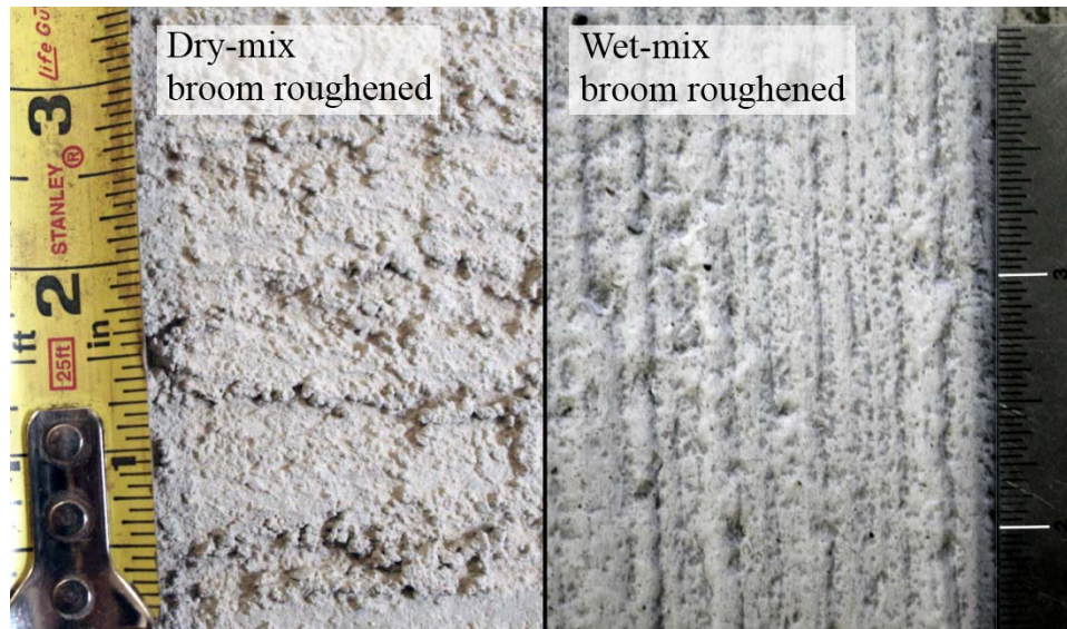
Figure 10. Visual appearance of dry-mix (left) and wet-mix broom roughened (right) surfaces.
