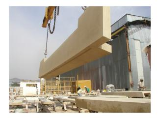
Real size mockups were made special for the Crescent building in order to check the geometry, right color, texture, dimensional measures, with "0" tolerance allowed.
