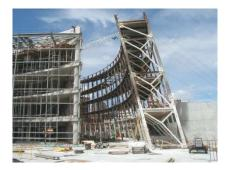
A total of 1,306 panels were required for in the Crescent building, 154 different panels at the outer crescent and 142 panels for the inner crescent elevation, with a total of 296 different panels with 24 different radiuses (concave, convex and warped) and several other vertical panels of the building as column covers.
