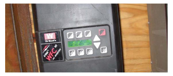
Photo 6: VFD at Load, 41 HZ or 15 feet per minute Note Load at 23% Plenty of Reserve Power
