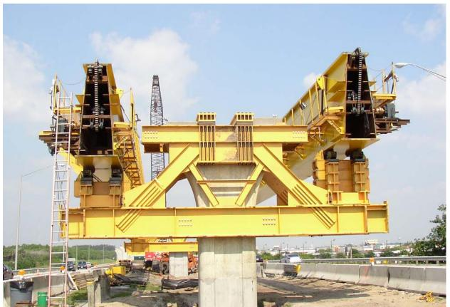
**Photo 1: Pier Bracket and Erection Girders**
