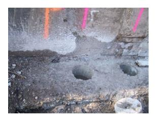
Fig. 8. (a) Holes Drilled in Existing Abutment Toe
