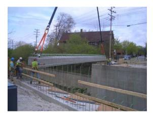
Fig. 14. (a) First Exterior Beam
