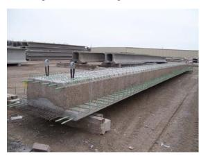
Fig. 13. (a) Completed Interior Beam
