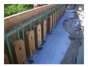
Fig. 17. (a) Forming Parapets
