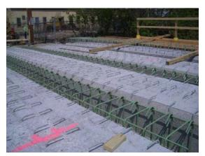
Fig. 16. (a) Slab Re-bar Cages Installed
