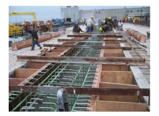
Fig. 12. (a) Forming Interior Beam
