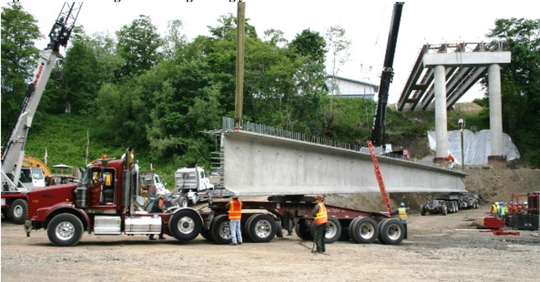
**Figure 7** WF-Series girder at bridge site
