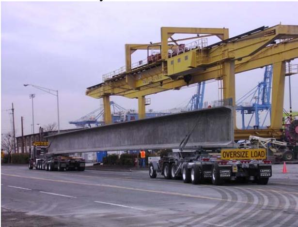
**Figure 6** WF-Series girder leaving casting yard
