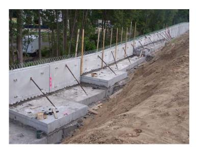
Figure 13. Bracing of Stem Segments
