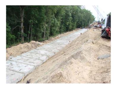
Figure 11. Erected Footing Segments of Wall A after Grouting
