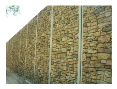
Figure 15. Finished Front Face of the Wall System with Aesthetic Treatment
