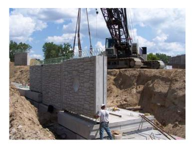
Figure 12. Erection of Short Stem Segments
