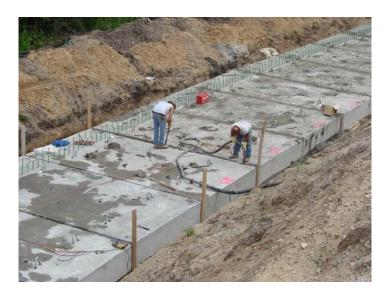
Figure 10. Grouting Operation for Footing Shear Keys
