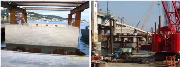
Fig. 5 Pier 3 Precast Cofferdam Cell
