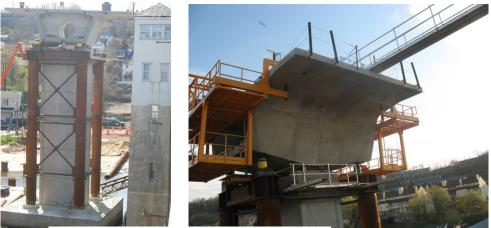
Fig. 8 Pier 3 Pier Table Construction
