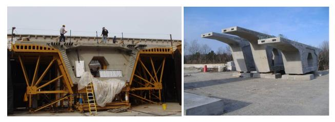
Fig. 6 Unistress Casting Yard: Segment Casting and Storage
