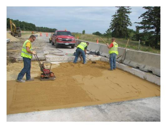
Figure 18 (Sand leveling surface preparation)
