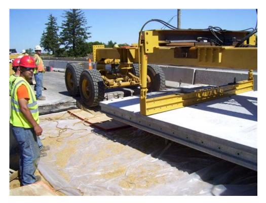
Figure 24 (Installation of panel using trailer transport)
