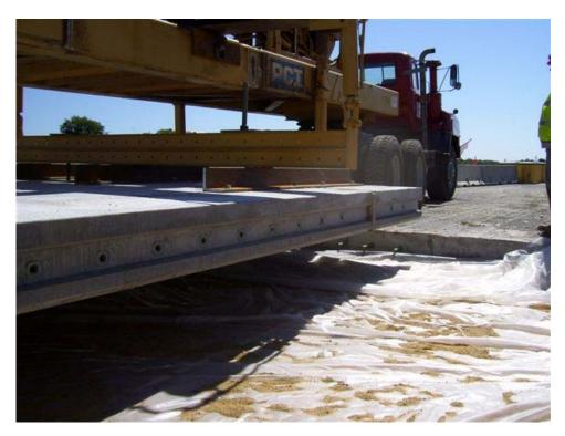
Figure 26 (Installation of panel using trailer transport)
