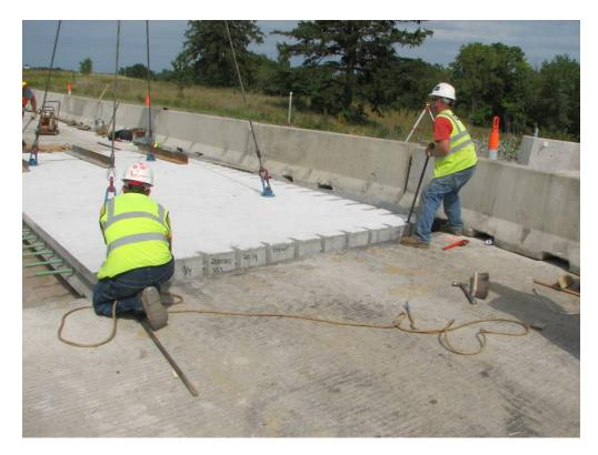
Figure 20 (Installation of first roadway panel)
