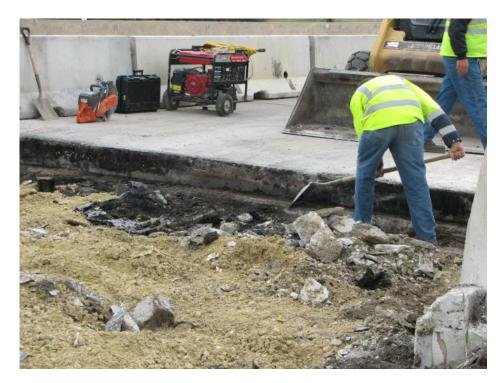
Figure 17 (Cleaning off existing paving notch location)
