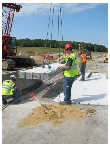
Figure 21 (Installation of inside 3'-10 shoulder panel)
