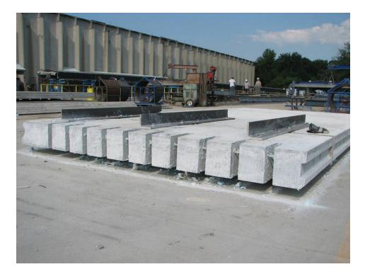
Figure 12 (12 ft Roadway panel in precasting yard)
