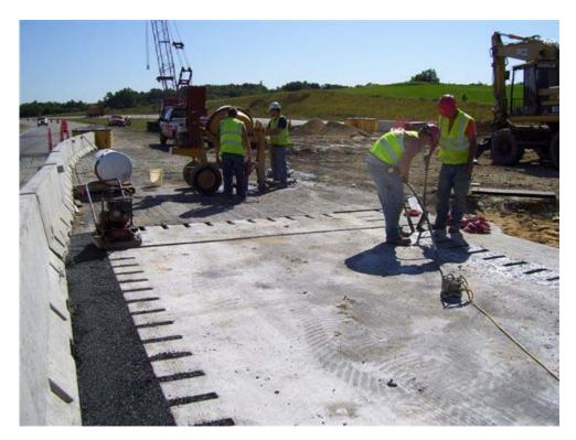
Figure 23 (Grouting pockets and temporary joint at centerline)
