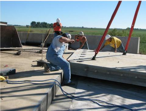
Figure No. 2 (Placement of First Panel at Abutment)
