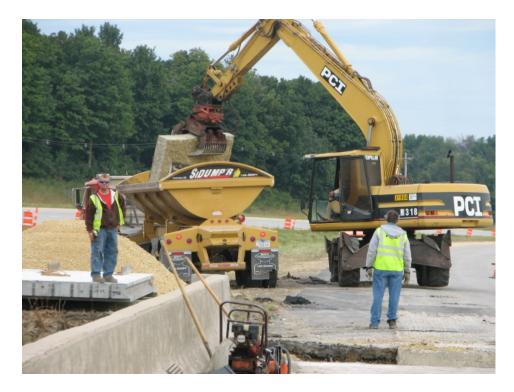
Figure 16 (Construction removing existing approach)
