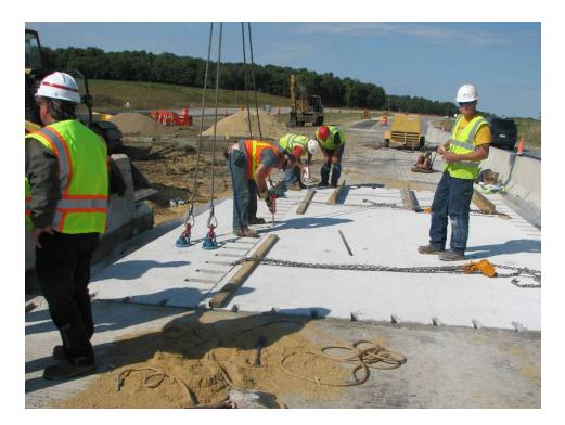
Figure 22 (Providing epoxy for keyway at shoulder line)
