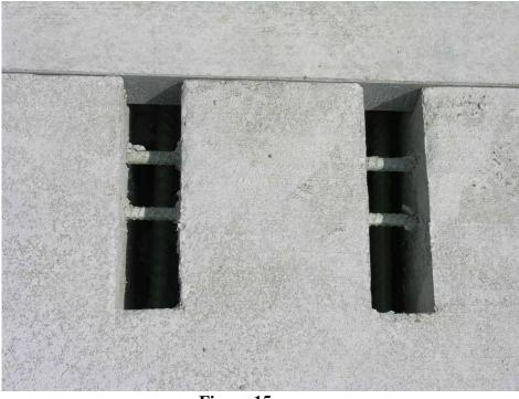
Figure 15 (Fit-up test at shoulder line showing pockets)
