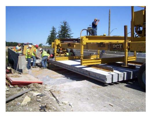
Figure 25 (Installation of panel using trailer transport)
