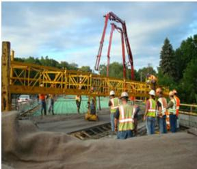
Lightweight aggregate sand (LWAS) provides water from the instant the concrete is mixed and the water comes into contact with the cement. High performance concrete with Internal curing is a curing method that provides a continuous application of water to the concrete mixture. The reasons are: (1) water is so fluid, (2) the capillary action is within the hydrating cement paste are so strong and (3) the thirst (water demand) of the cement is so intense.
