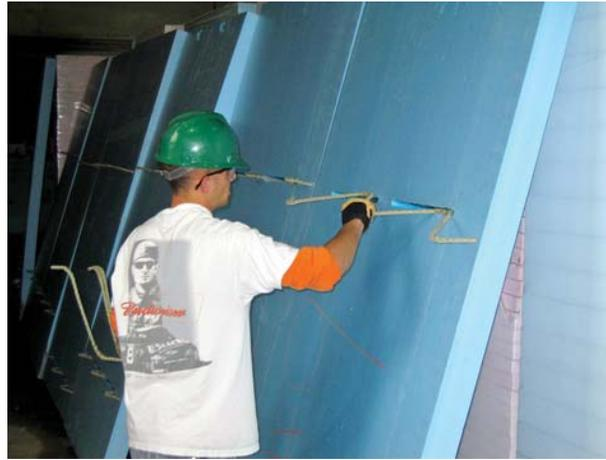
Fig. 5: Inserting NU-Ties in the slots of the EPS panels
