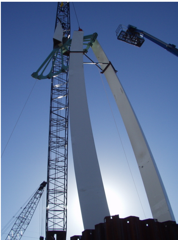
Fig. 2 Erection of steel tower legs
