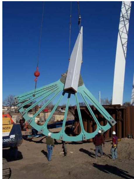
Fig. 7 Upper Cable Anchorage Assembly & Tower Top
