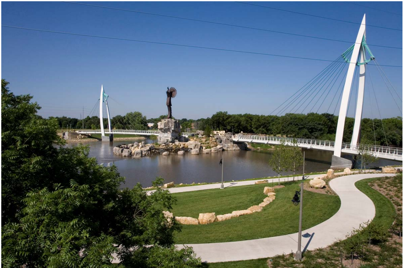
Fig. 9 Completed Pedestrian Bridges
