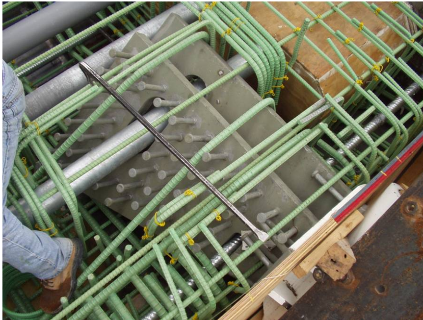
Fig. 6 Lower Cable Anchorage Plate placement
